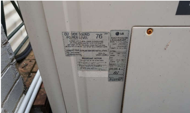
Photograph 13: Split air conditioning unit containing R22 refrigerant gas.
